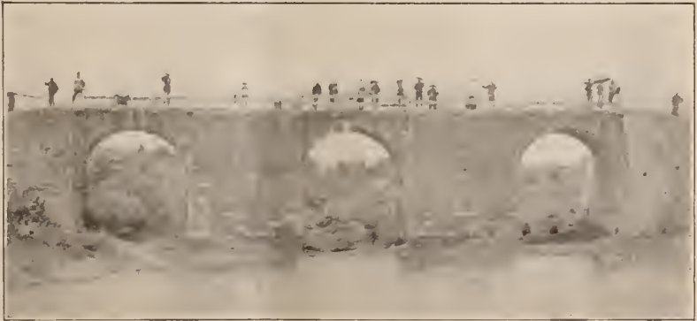
BEST BRIDGE IN HAINAN, CHINA.
